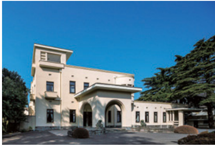
本館外観 Exterior of the Main Building
